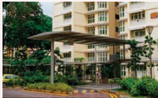
b) After upgrading: An additional study cum utility room for each flat and a drop-off porch for the block
